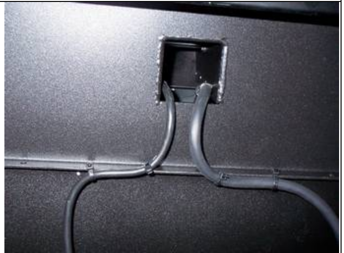
Figure 9. Cables are secured in the rear with tie wraps.
